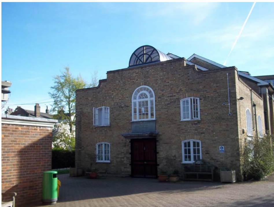
View from within the site showing front of Founders Hall
