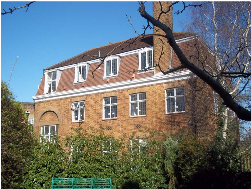
View from within the site showing rear elevation of Elizabeth House
