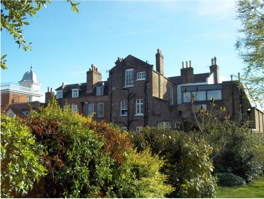
View from within the site showing rear elevation of 108-112 The Bank
